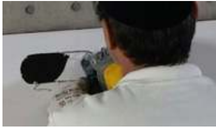
b. Use a jig saw (tool 6) to cut through the panel
