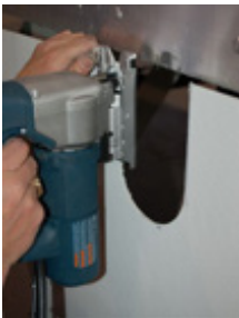
a. Use a 4 1/2" hole saw to make a round opening for the tank nozzle. It is possible to make a "U" shaped opening if considered easier for the driver to access the nozzle.
